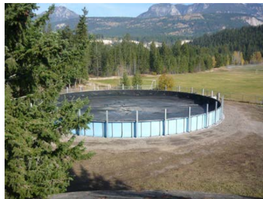
Hypalon Reservoir Liner Replacement Planning
