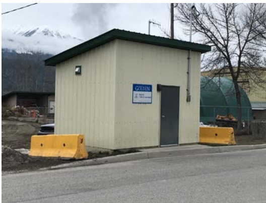
Well 4 Structure Replacement
